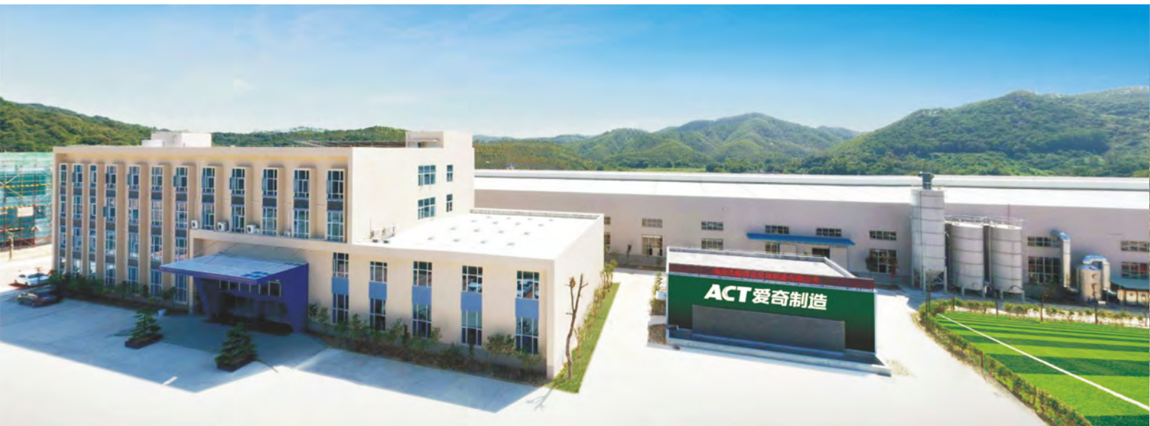
ACT Guangdong Manufacturing Base
