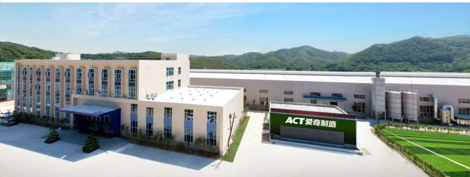
ACT Guangzhou Manufacturing Base (Area : 100,000 m 2 )
